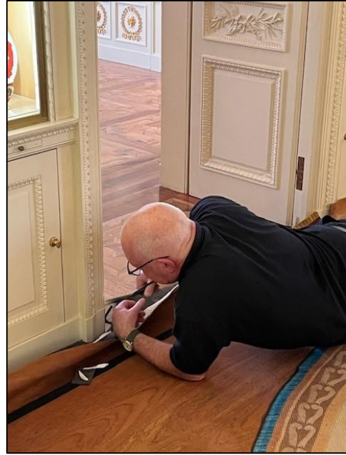
Figure 8. Custom cutting the Eyemats and the Egalsoft backing to accommodate the Icon Room doorway.
