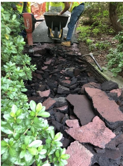
Demolition of the paths
