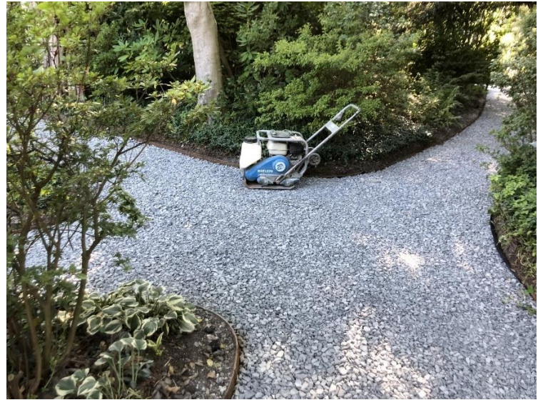
The newly compacted gravel
