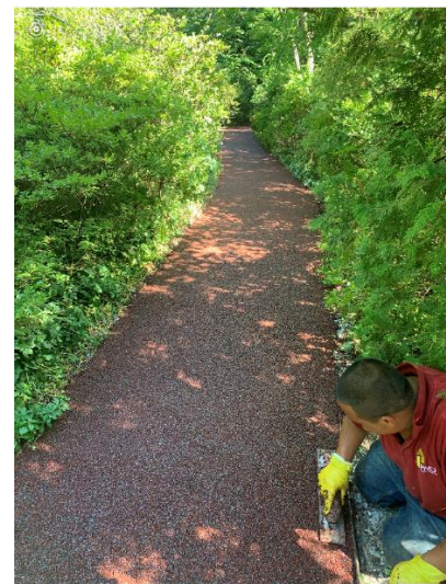
A team member spreading the paving material
