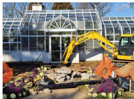
Water main repair in front of the greenhouse entrance
