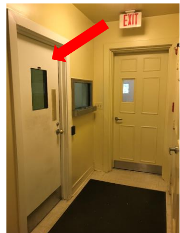
Mansion Security Control Room
