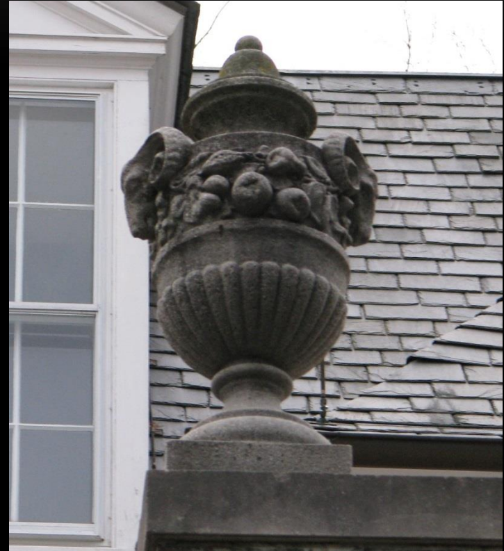
Urns On top of Porte cochere
