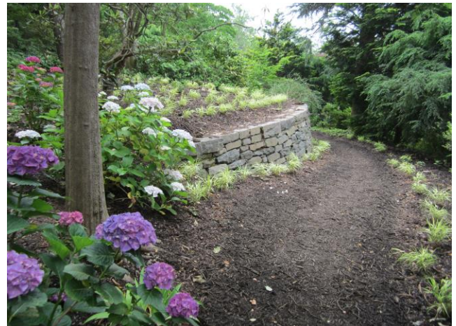
Retaining wall original to Marjorie Post's residence
