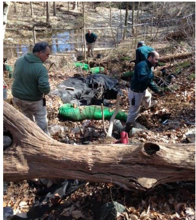
Staff installing shrubs to reduce erosion
