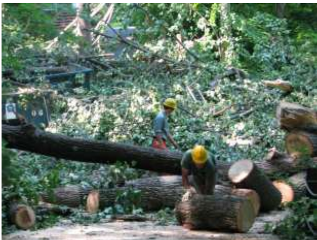
Davey Tree helping cut and remove fallen tree branches
